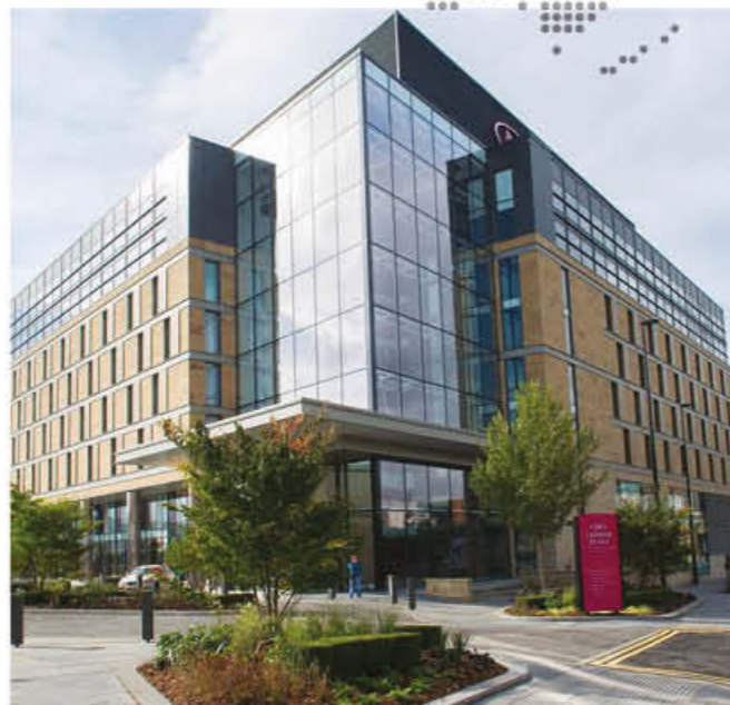
Hotel built using off-site manufactured pods
